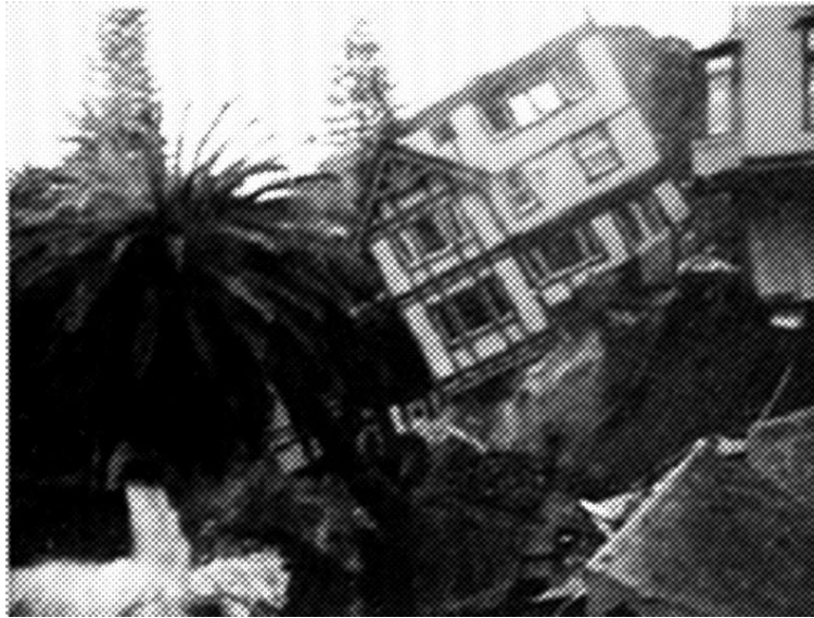
A sinkhole caused major damage on Dec. 11, 1995
